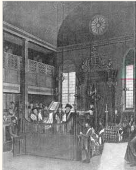
Interior of a Synagogue in Portsmouth
